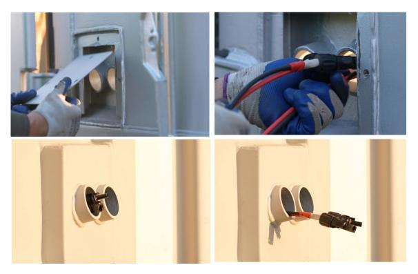
Take off the cable hole cover on the side door of the container, and route the PV DC cable through the cable hole(The right hole is used to route DC cables, and the left hole is used to route AC cables)
