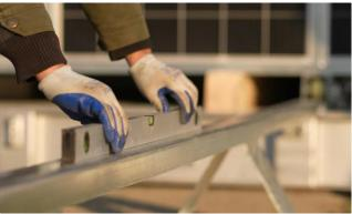
Make sure that the two tracks near the container are of the same height(The level bubble should be in the middle)
