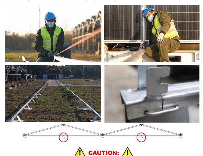
Track support must be placed in the middle of the single track
