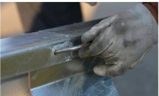
After all the tracks are installed, the flatness of the tracks is calibrated by drawing straight lines; Place two Track stops at the opposite end of the container on the last Track supports. Secure the Track stops by inserting a U-screw.
